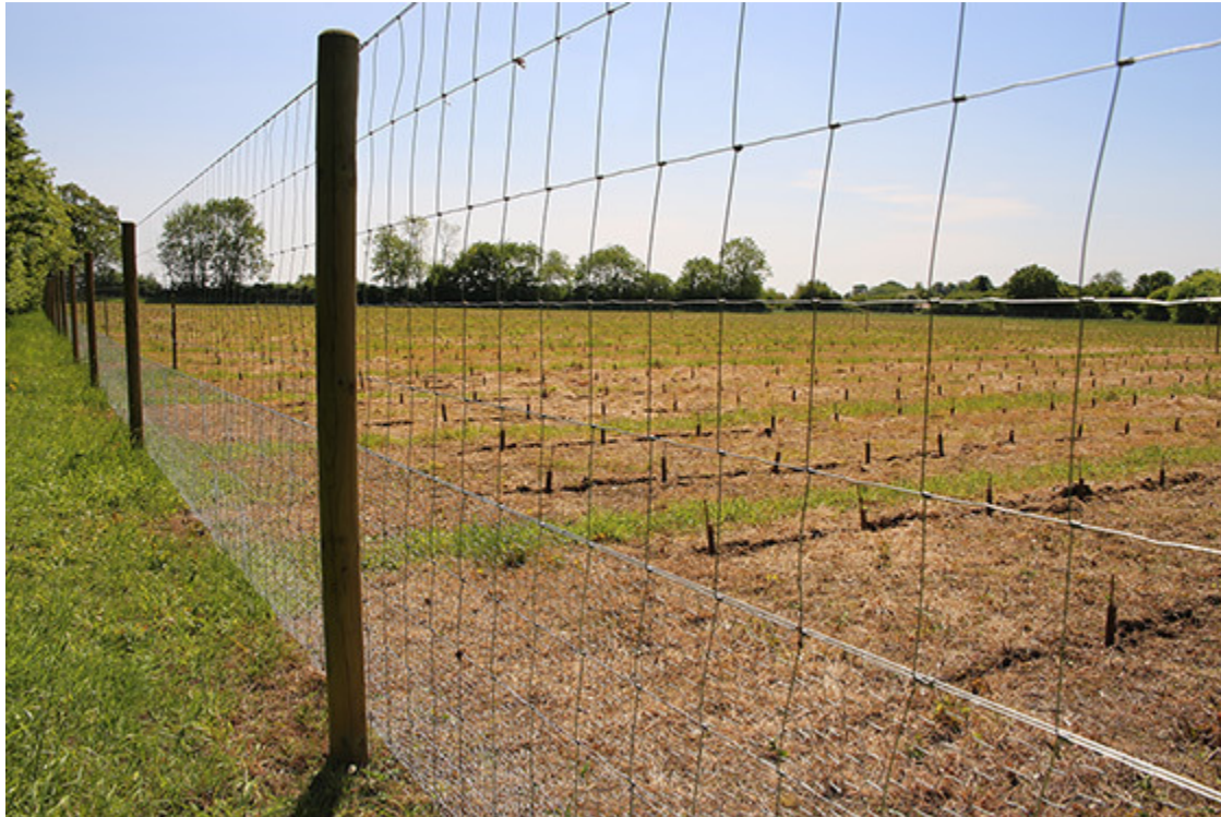
Working with the Forestry Commission on ash dieback recovery schemes has created some large clearance and fencing projects for Paul and his team. Pictured is fencing to keep animals including deer and rabbits out of one of the young tree plantations in mid-Suffolk.
