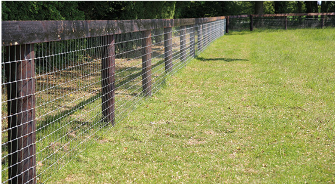
Recently-installed stud fencing.
